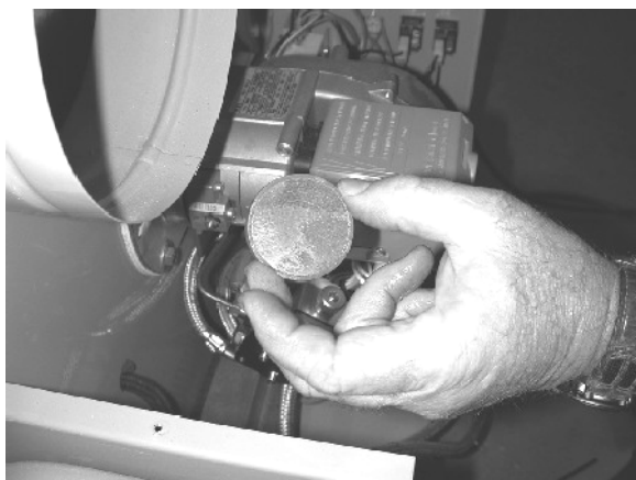
Remove the fuel pump screen
