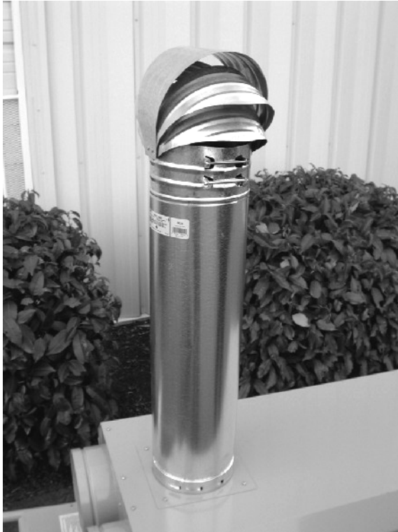
Attach the flue to the Dragon
